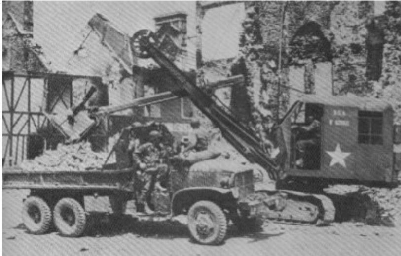
**Figure 3: Mechanical Earth-Moving Equipment – Using Cables To Transmit Loads**
