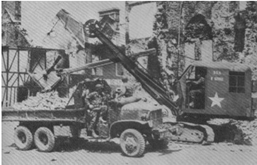
Figure 4: Mechanical Earth-Moving Equipment – Using Cables To Transmit Loads
